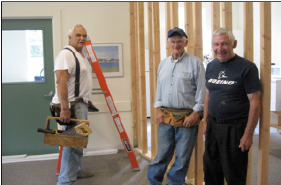
Bill Shain, Ken Winter and Larry Elton built the double-wall partition in the background.
