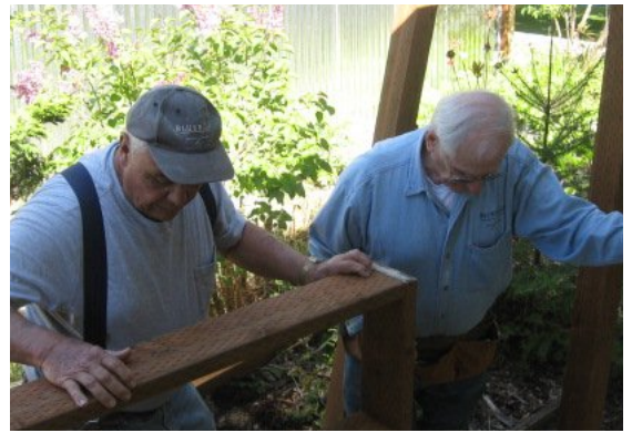
Bill Shain and Ken Winter work on getting the upper landing installed.
