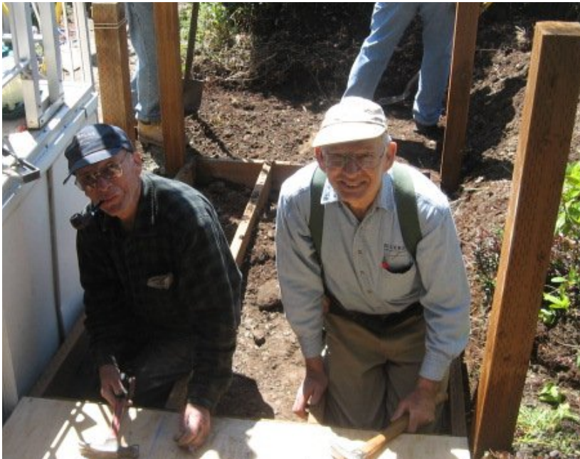
Giff and Ken nailing down plywood flooring.
