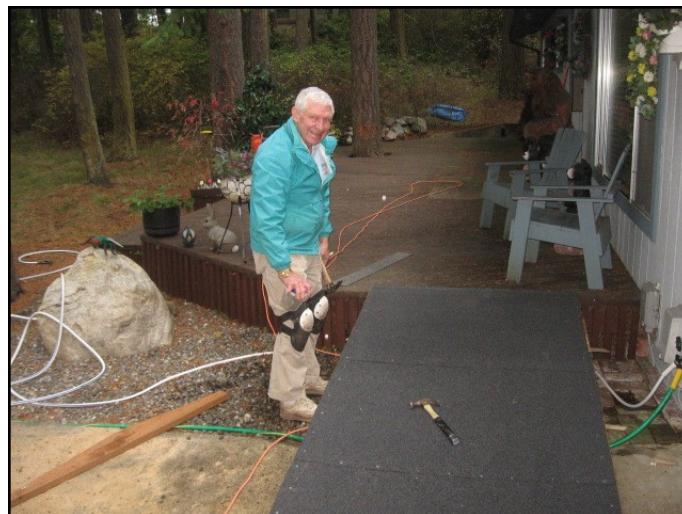
Larry has just finished nailing down the roofing. Some old OSB provided by the client was used in place of plywood. We covered the entire surface with roofing to give it a little more durability.
