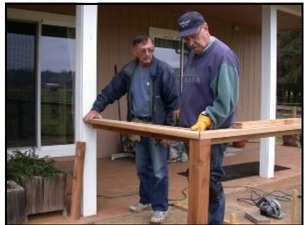
Doug Rittenhouse and Ken Orth check railing fit.
