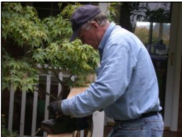
Rod Harp uses a belt sander to put the final touches on a railing.
