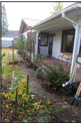
Area where ramp will be built.
