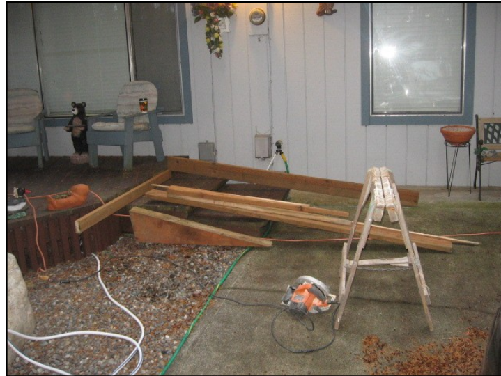
The job site. The ramp was build over the existing steps.
