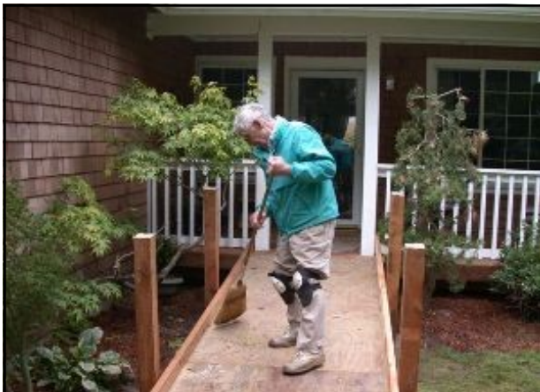
Larry Elton sweeps up prior to installation of the roofing material.
