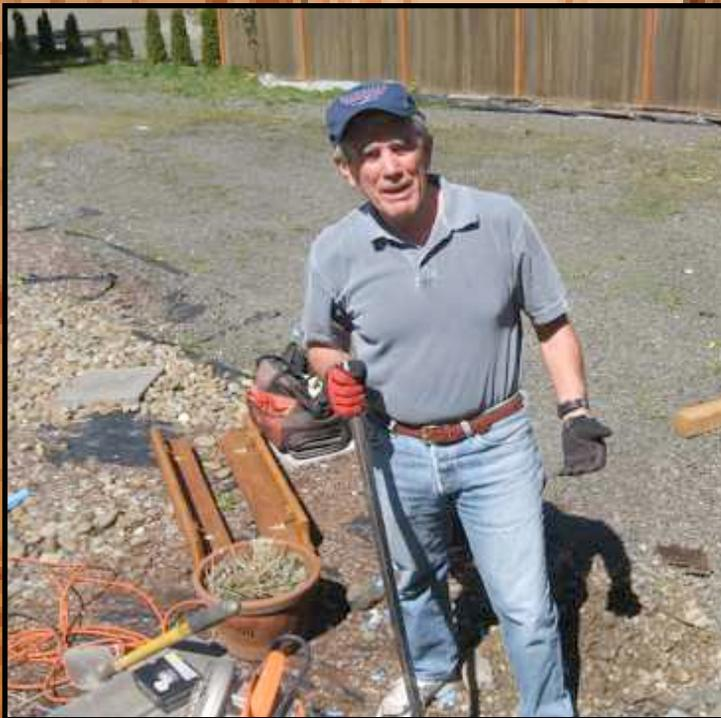
**Ed Berthiaume digs a hole one of the 4x4 posts that will be used to support the handrail. Lots of gravel and large rock to work through.**
