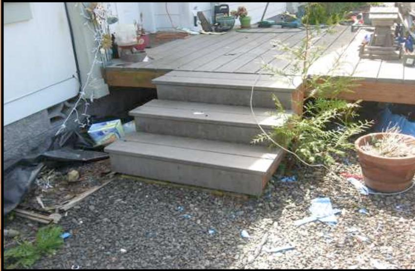
**This set of steps is a typical problem. The porch is low enough That the building code doesn't require handrails. Elderly or Disabled can find the absence of handrails real difficulty or danger.**
