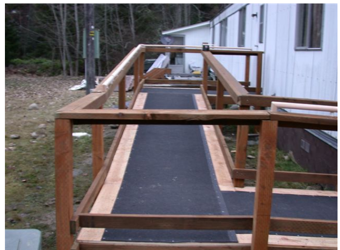
The finished ramp.
