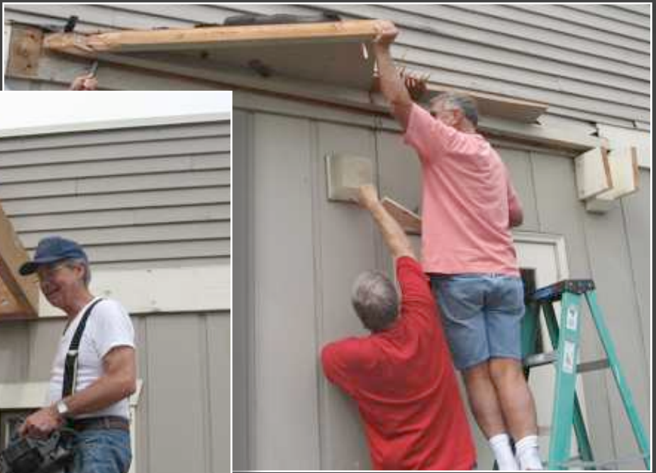
Jack Hawker and Mike McFadden dismantle an overhang to make way for the new beams.
