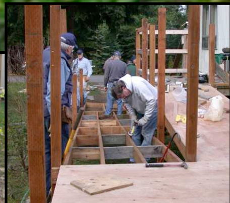
Marv and Mike attaching ramp joists to the support posts.
