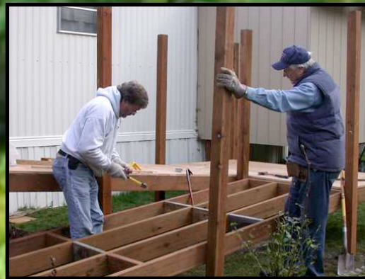
Marv and Mike attaching ramp joists to the support posts.
