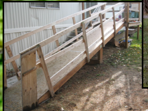
The existing ramp was too steep for the user to get up and difficult to get down. The slope on this is about 4/1 (four inches of "run" for every inch of "rise"). The building code and Bluebill specification call for a minimum of 12/1. The old ramp was removed during the rebuild.
