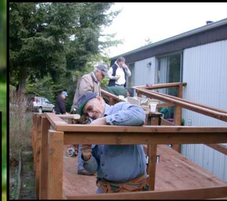
Mike Mallett and Marv Segar install support posts.
