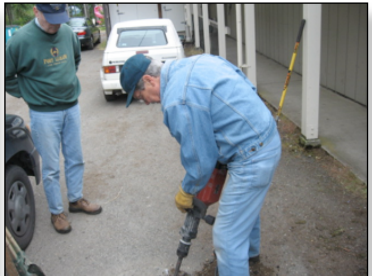
Chuck Sherrard uses a jackhammer to dig footing holes. Dick Gildeen looks on. The holes are two feet deep and one foot in diameter.
