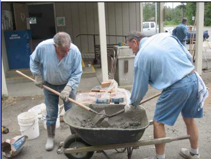
Jack Hawker and Steve Failla fill one of the footing holes with concrete
