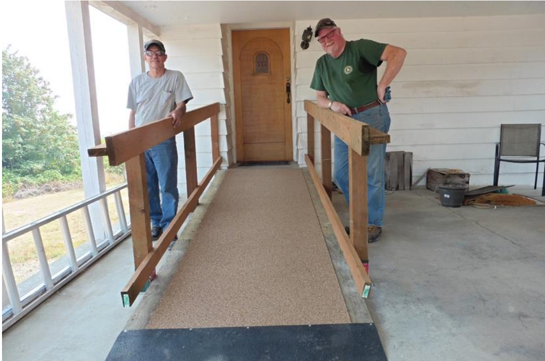
Bob Keever and Wally Grenquist with Newly Installed Ramp
