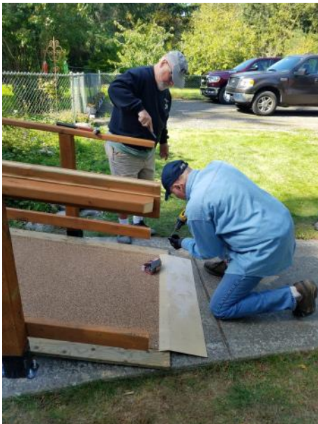
Richard smoothing the edges and John installing the threshold.
