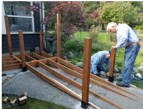
John and Joe anchoring post to the sidewalk.
