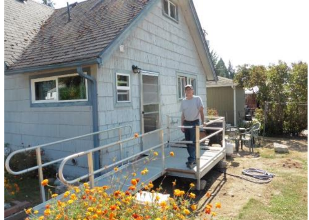
Installed Platform with 8' Ramp (Bob Keever)
