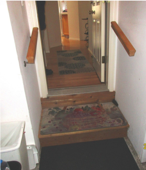
The steps from the garage into the house. It would be difficult to navigate these in a wheeled walker.
