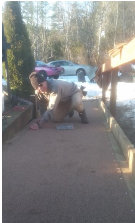
Richard Knapp Nailing Down the Mineral Roll Flooring
