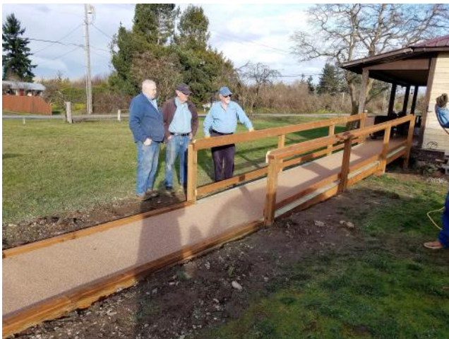
Another Clallam Co. Ramp build
