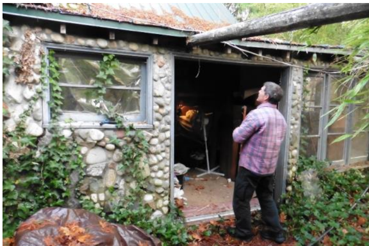
Bedroom wall before repair
