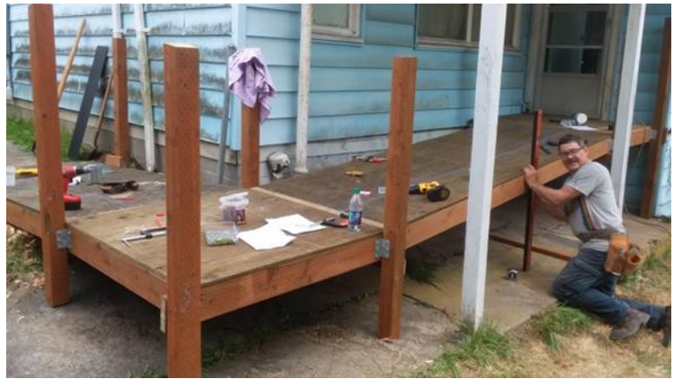
Master Builder, Greg DeVault, keeping things in check
