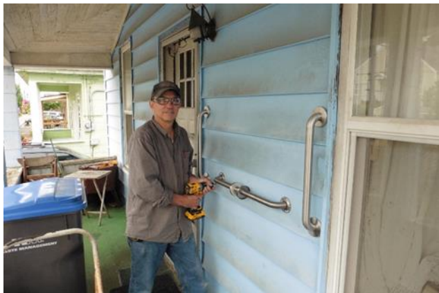
Bob Keever installing grab bars.
