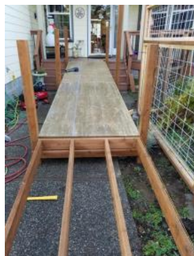
The decking goes down.
