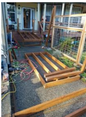
Framing Partially Complete.
