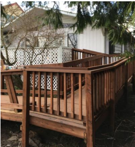
Completed picture of the 2 ramp. 2 platform "tricky bit".
