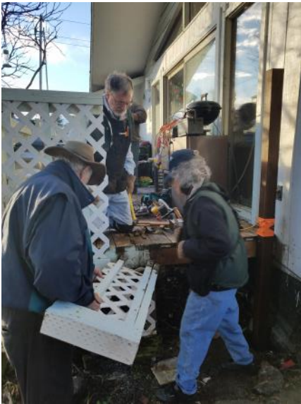
Michael, Dan and Jo begin demolition.
