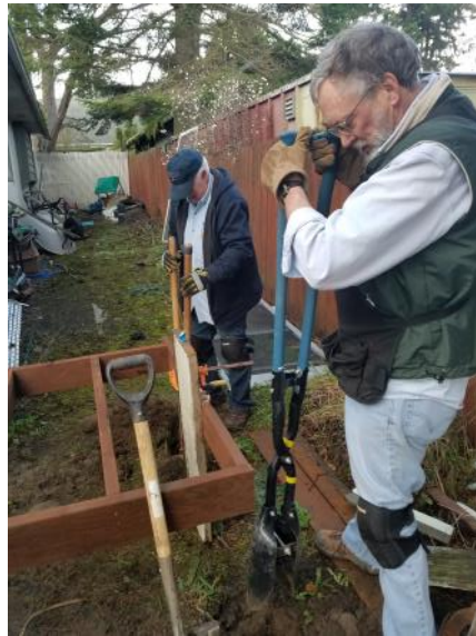
Dave and Dan working on two of the many postholes.
