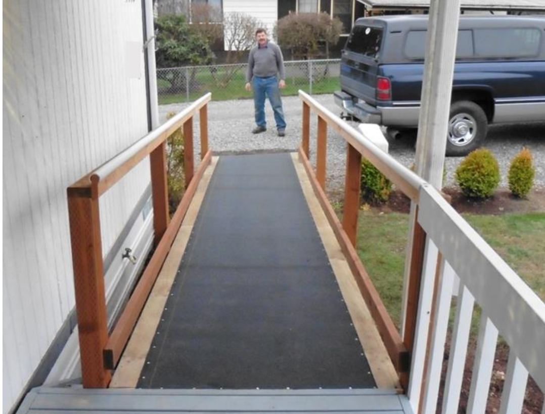
Greg DeVault at the bottom of the newly installed ramp
