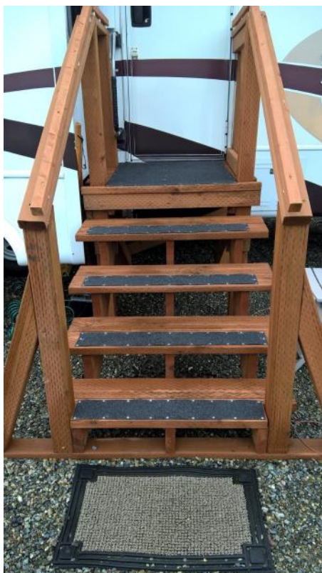
This client was complaining that her steps were slippery. Robert Chanpong nailed down some roofing.
