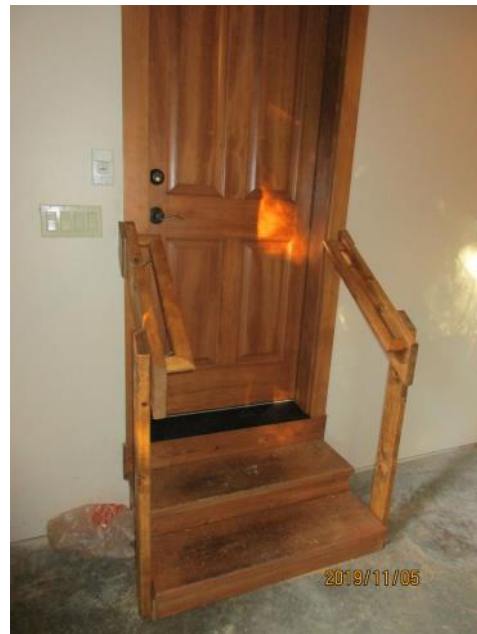
Railings installed on both sides of steps.
