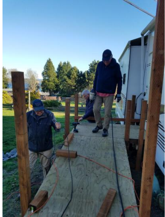
Trimming the posts and installing the kick rail. Myron Vogt, Joe Gagnier, and Rick Morasco.
