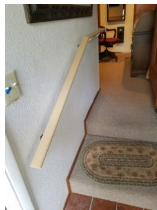
Handrails installed up the steps and around the wall take over when the client has to leave her walker at the bottom of the steps.
