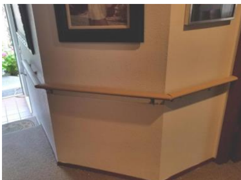
Handrails installed up the steps and around the wall take over when the client has to leave her walker at the bottom of the steps.
