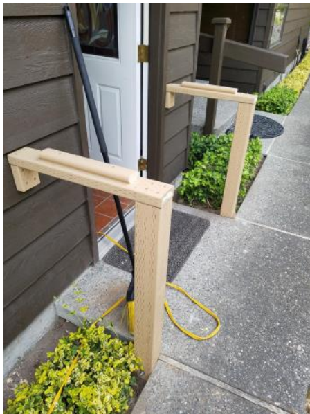
New handrails to the garage door. The railing previously installed is in the background.
