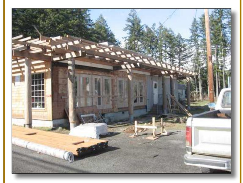
Work is currently in progress on the door-side wall. There will be a 16 foot deck running from the corner to the step shown in the picture. Footings for the deck are ready for pouring. Ultimately the entire wall will be shingled to match the front.
