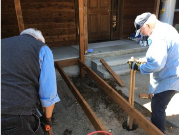
Michael Graham and Dave Parish digging post holes.
